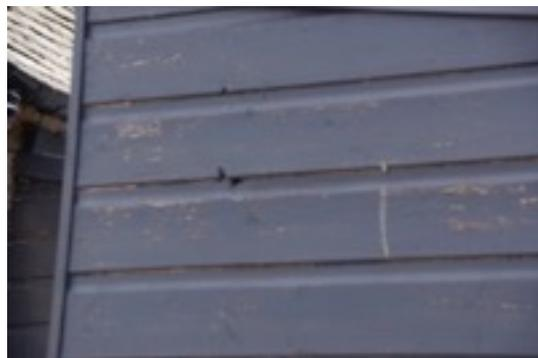
External paint on the entrance to the drop-in in very poor condition with signs of minor signs of wet rot, clear evidence that wood was not properly prepared during initial work. Paint on the rest of the drop-in and store beginning to show signs of stress and need of a new topcoat. Paint on the boiler house beginning to weather, there is a need to apply a new topcoat.
