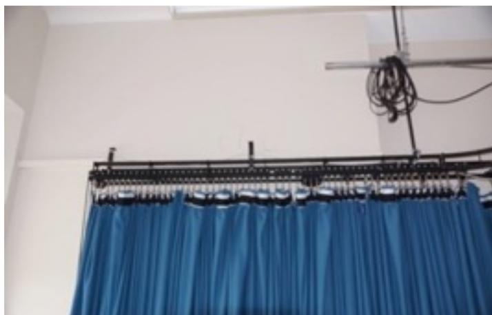
Curtain support to the west in the blue room has moved from the wall and requires to be secured.
