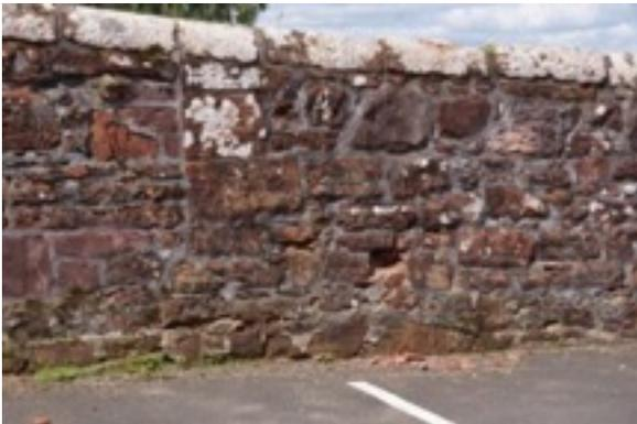
Boundary wall deteriorating badly, could become dangerous
