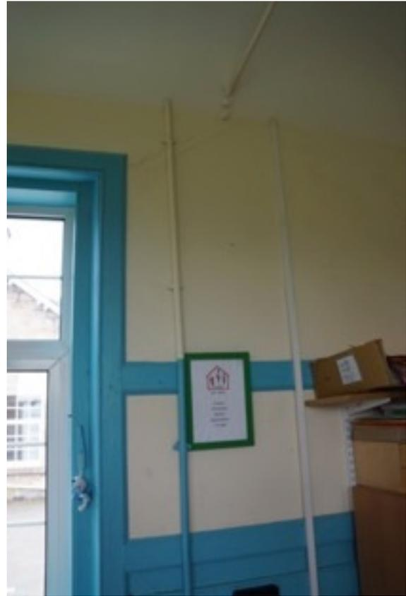
New window surrounds require to be knotted and primed. All redundant ducting, wiring, wood straps and metal requires to be removed and surfaces made good.
