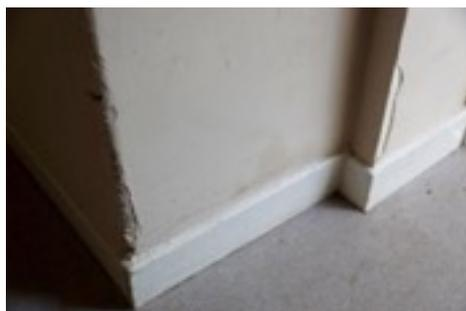
Various holes and broken plaster require to be patched
