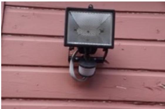
External lights causing main board to trip, also at drop in they are not in a location the illuminates the key box and entrance.
